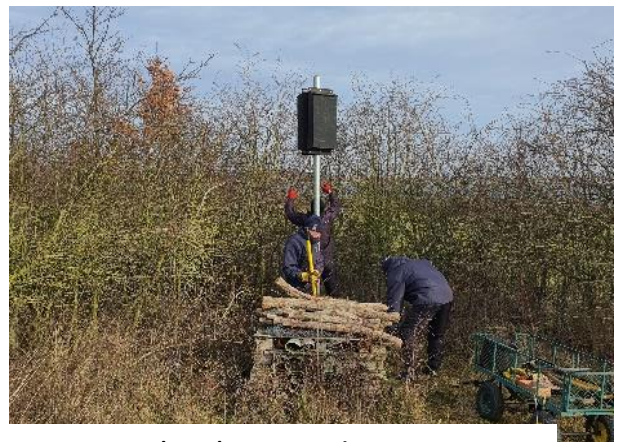
Bat pole under construction
