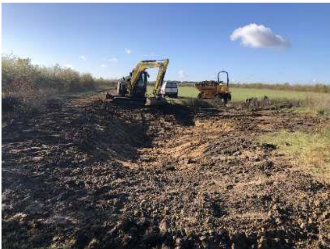
New Mitigation Pond being created
