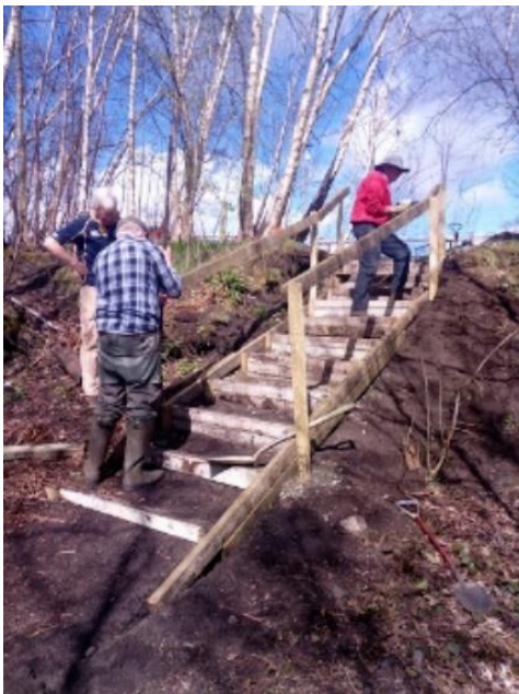
New steps being installed by volunteers
