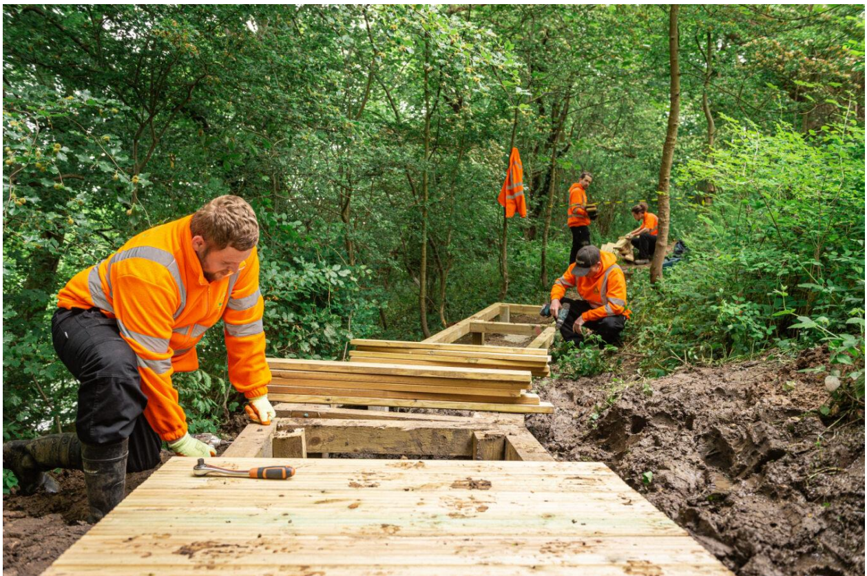
Boardwalk under construction by trainee Wardens
