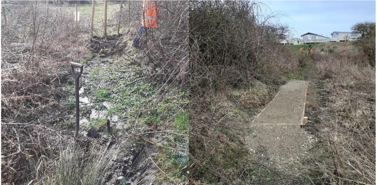
Footpath improvements, Sandy Bay
