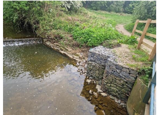
New seating provided / restoration of existing seating areas / revetment work for bridge
