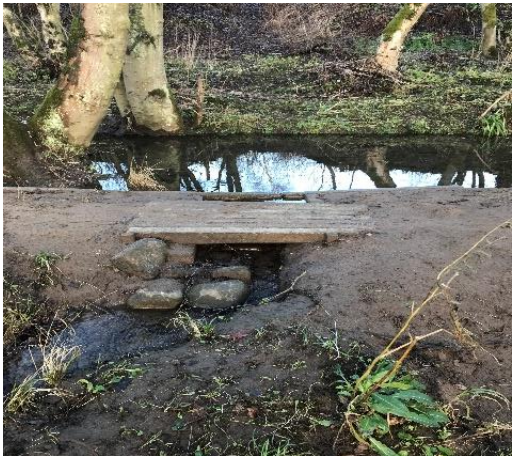
New pond with a leaky dam outlet
