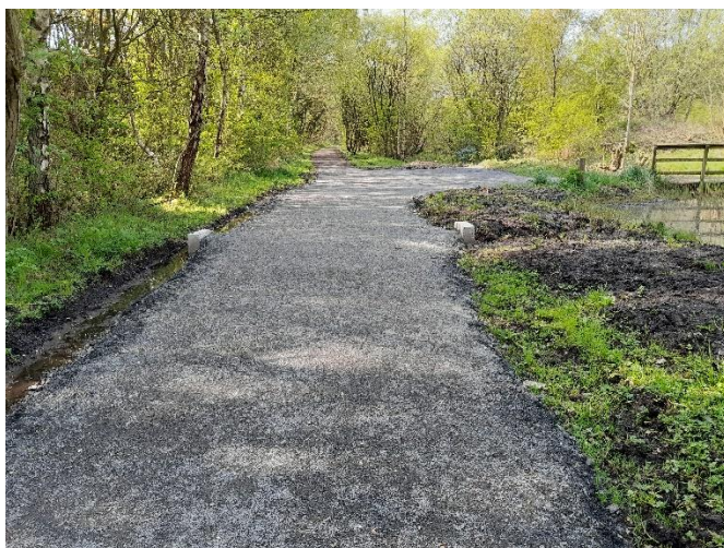
Path surfacing improvements with improved drainage
