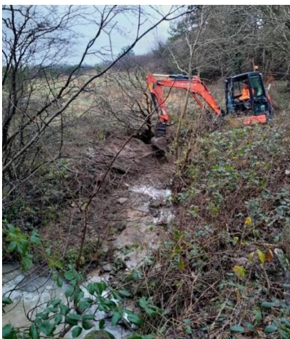
Overflow channel construction
