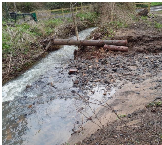
Overflow channel after heavy rain
